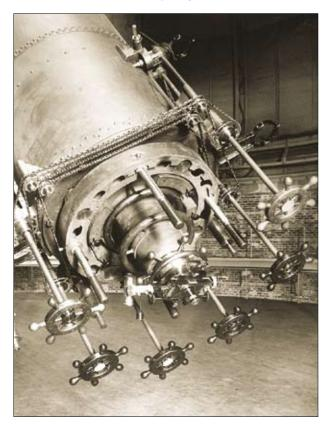
**Figure 7** Eye end of the Yerkes 40-inch refractor shows all the knobs for operating the geared rods that controlled the telescope's motions—a major improvement Warner and Swasey made to telescope design.
