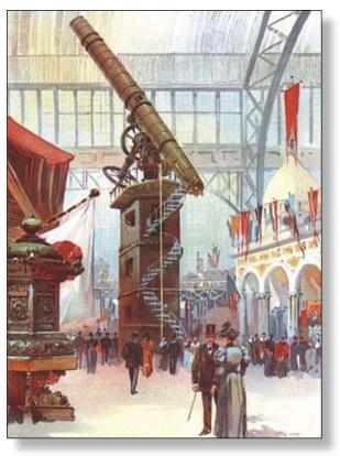
Figure 6 The second world's largest built by Warner and Swasey was the 40-inch refractor for the Yerkes Observatory of the University of Chicago, here displayed at the Columbian Exposition in Chicago in 1893. Despite its many similarities to the Lick 3-inch, one major advance was the electrical system for controlling the telescope's motions. It remains the world's largest refractor.
